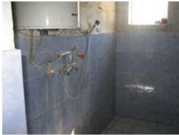
Electrical wiring in the bathroom is short of minimal safety standards and is dangerous for people there.
