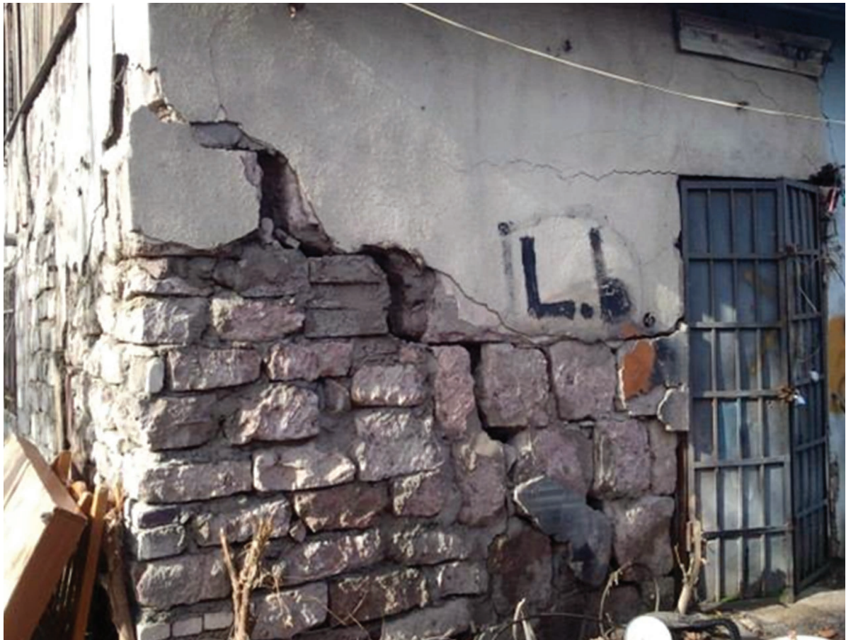
Building of Sakinformagroprom, Ketevan Tsamebuli st. 71, Tbilisi
