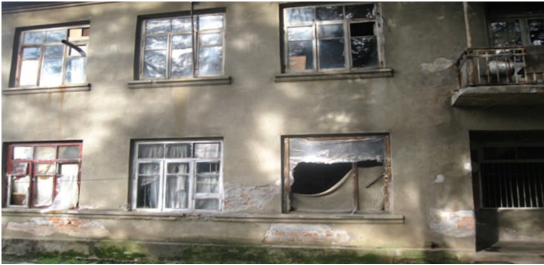
Zugdidi regional hospital building.
